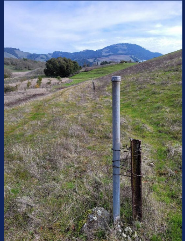
Matanzas Dam - Downstream Stability Berm (Facing North)
